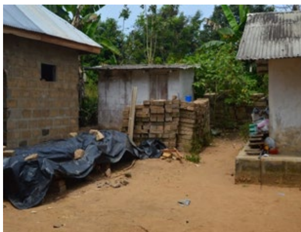
Existing Church at Ehoaka
